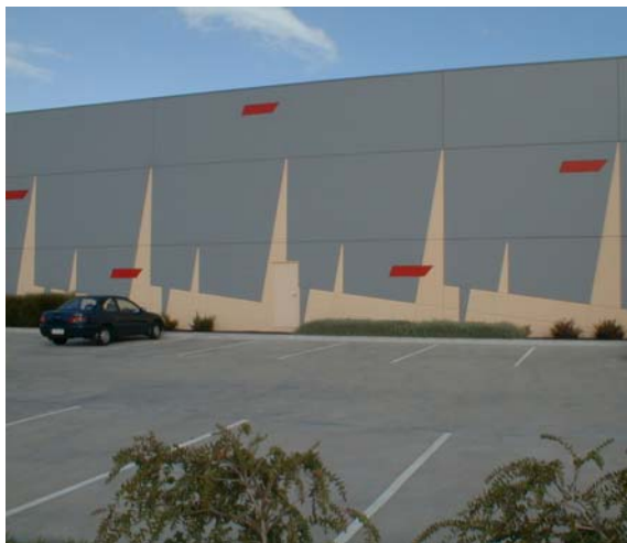
Feature tilt-up panel design incorporating Premium-flex joint sealants.
